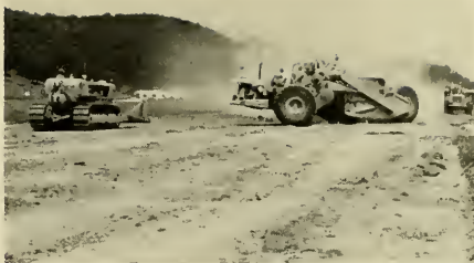
HEAVY EQUIPMENT prepares the base for Ohio University's hard surface runway which has been scheduled for completion the first of October.
